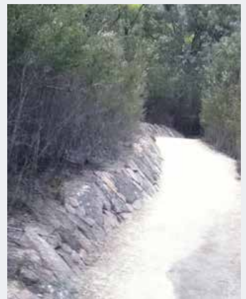
Bench-cut contour tracks have a gentle crossfall that results in water draining off the track in thin, dispersed sheets rather than along the track.
