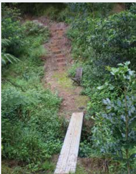
These basic steps traverse a steep slope down to a creek that is undergoing revegetation. Two trestle-planks welded together make a simple bridge.
