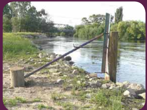
A flood-proof fence on the Murray River. This fence has survived several floods unharmed.
