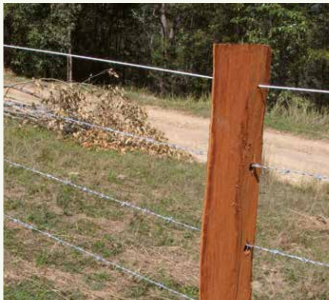
A top strand of plain wire or borderline (as shown) will help reduce wildlife entanglements and is strongly recommended in high risk sites such as around dams, on flight paths and along ridgelines. Borderline is a high-tension nylon wire that is both strong and highly visible. Photo by Sylvia Hood.
