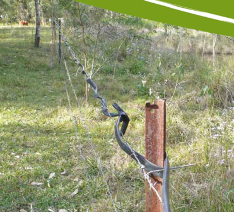
Wrapping old irrigation polypipe around the top strand of a barbed wire fence can help reduce wildlife entanglements, especially in high risk areas such as around this dam.
