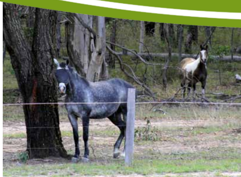
A simple hardwood post and three strand plain wire fence is friendly to both wildlife and domestic animals.
