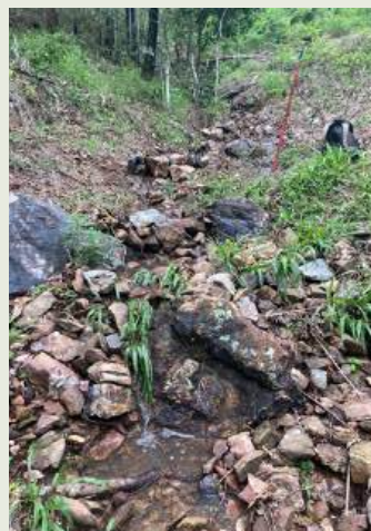
Rocky silt traps reduce the water flow energy and trap silt, enabling plants like lomandras to become established.
