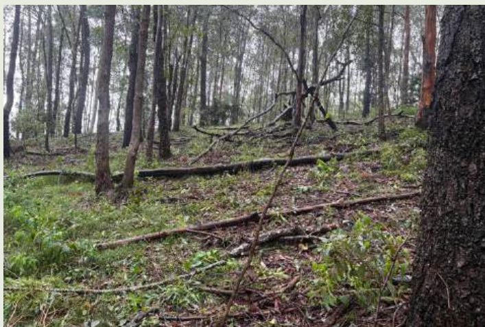
Logs and branches have been placed across the slope to slow surface run-off and trap sediment and encourage plants to grow.
