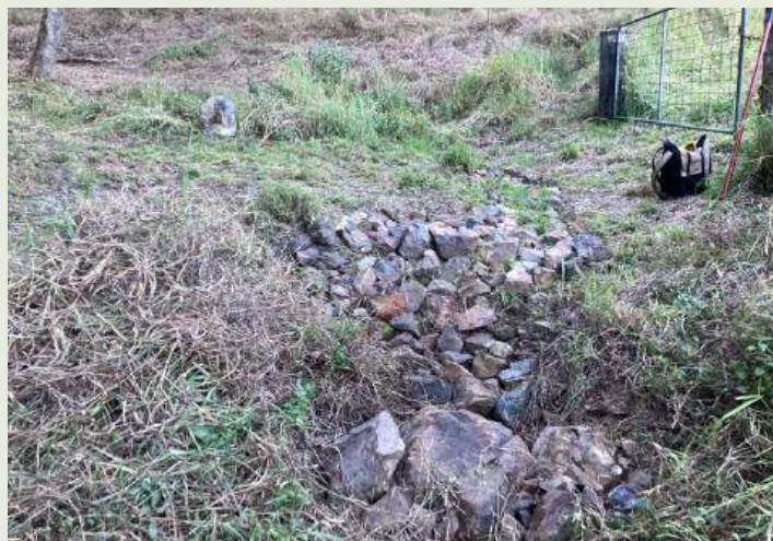
Rock flumes reduce the energy of flowing water.
