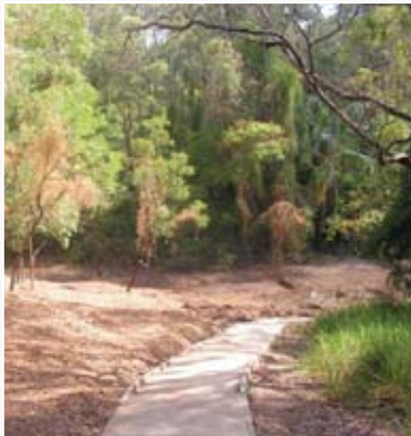
Site 1 at Finney's Hill - during restoration - getting the site ready for revegetation.
