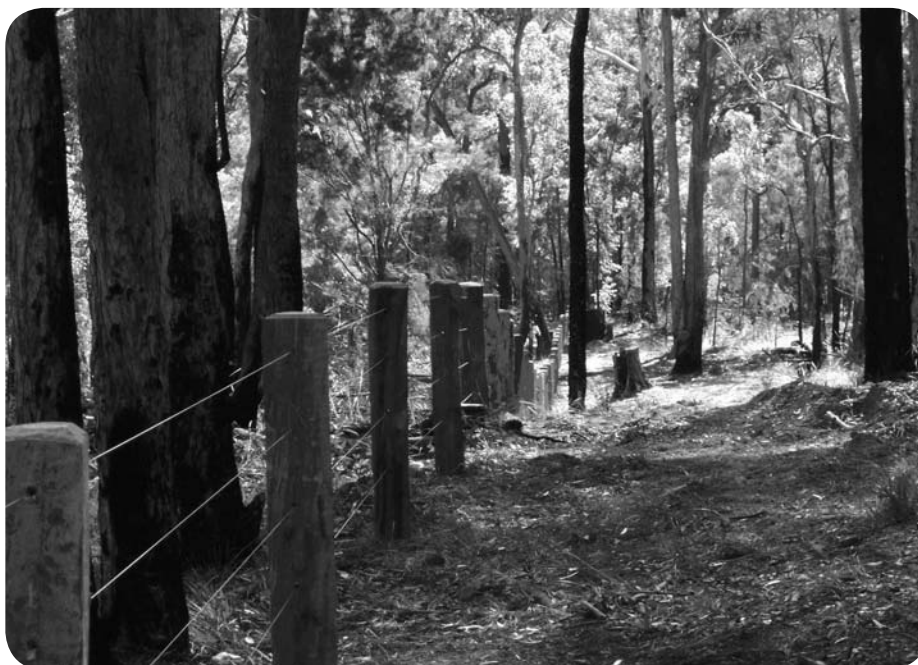
A simple hardwood post and 4 strand plain wire wildlife friendly fence.
