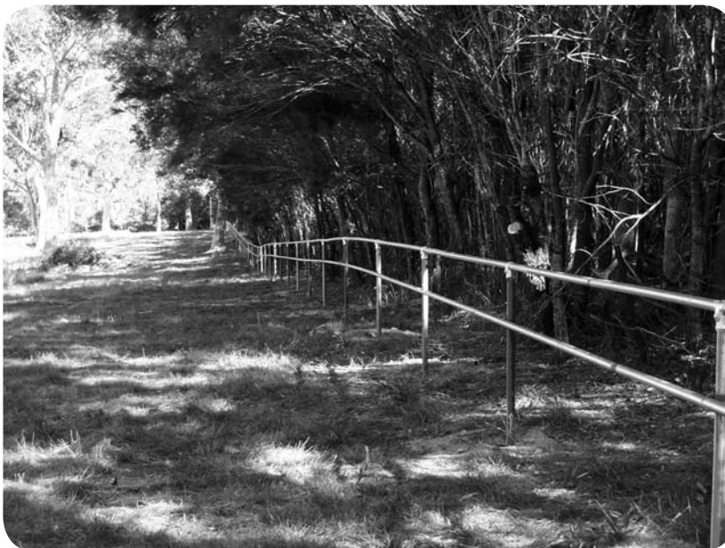
The after shot of the above box mesh fence line. It has been replaced with a galvanized pipe fence with a clearance of 75 cm from the ground level to the first pipe. The fence serves the dual purpose of being wildlife friendly while containing the owner's horses.
